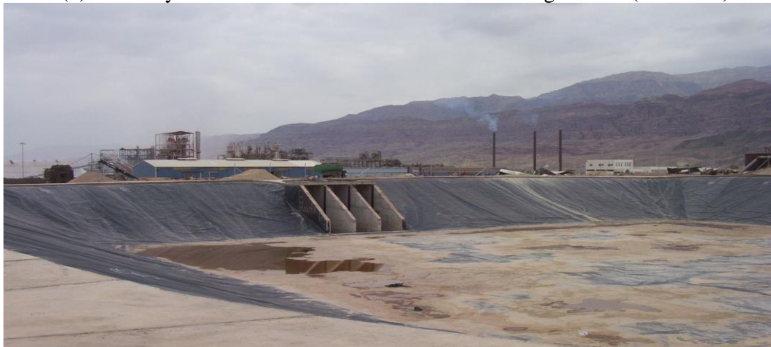
Photo (4): Refinery Collection Pond For Sub-Surface Drainage Water (side view)
