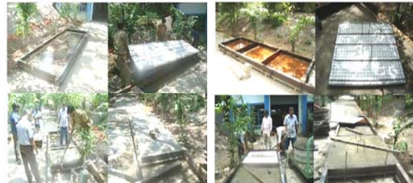
Figure 3. Casting of 3D sandwich wall panel
