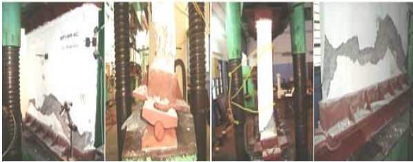
Figure 16. Figure showing failure of WP1-AC
