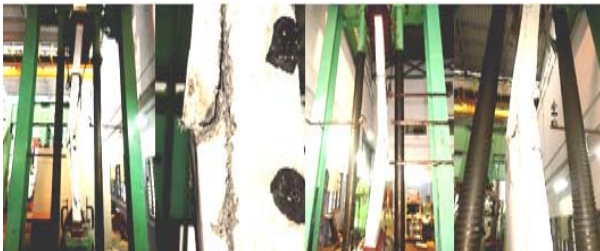
Figure 17. Figure showing failure of WP2-WR-AC
